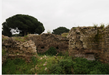
A view of east side before restoration works
