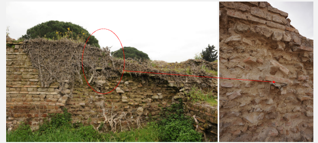
Stems wood of ivy plants, climbing with adventitious roots, are one of the main conservative problems in the site. The restoring treatment included its gradual cutting and removal
