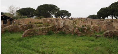
A view of west side before restoration work
